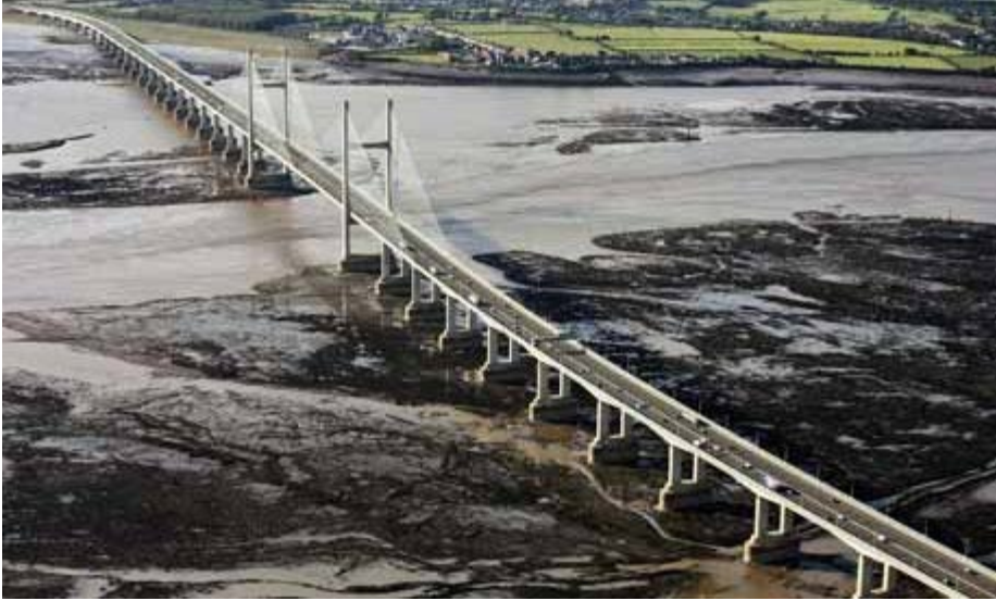
Aerial view of the Severn crossing. Photograph: David Goddard/Getty Images
